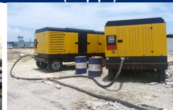
Pressure Test (oil pipe)
